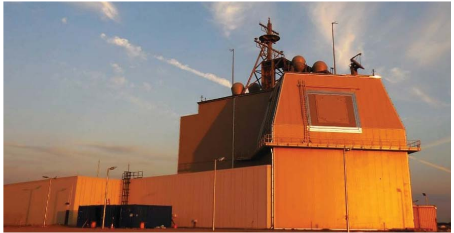
Aegis Ashore Deckhouse Deveselu, Romania
