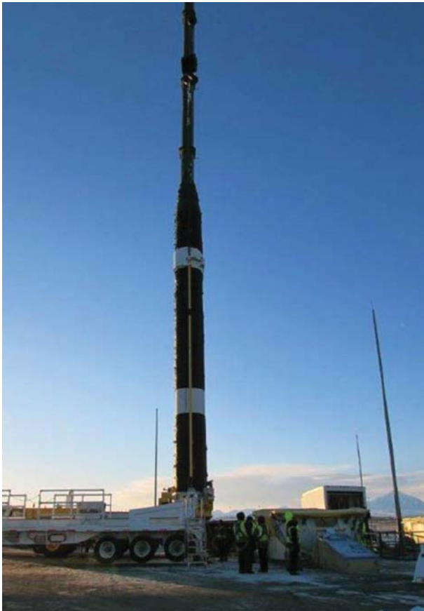
Ground Based Interceptor Emplacement Fort Greely, Alaska
