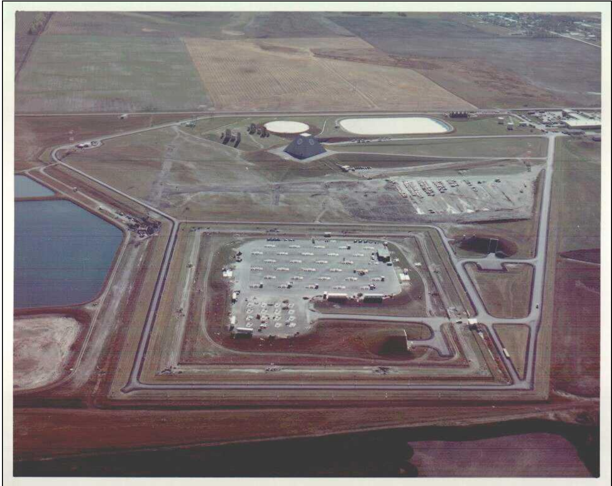
Aerial View of Completed MSR Site (Courtesy US Army)
